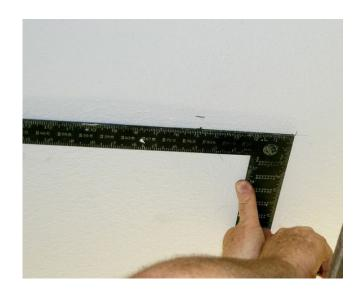
Use a square to align the first track to be installed.
