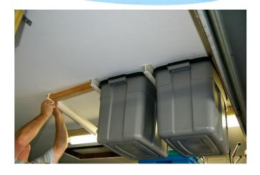
Subsequent track installation can be made easy by cutting a piece of lumber to use as a spacing guide. Note that the lumber should be cut ¼" under the desired track centers. In case of a 16" OC spacing the wood is cut at 15¾".
